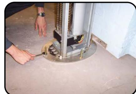
Using a hacksaw carefully cut the projecting bolt flush with the nut, ensuring the base plate is not damaged or marked in any way.
