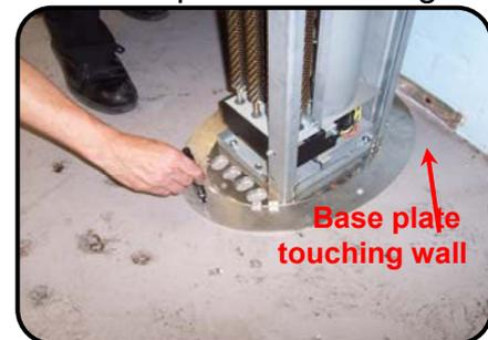
Reposition the air curtain base plate over the projecting bolts. Tighten each M10 nut as indicated in the adjacent picture. Ensure the vertical unit is secure, level and square.
