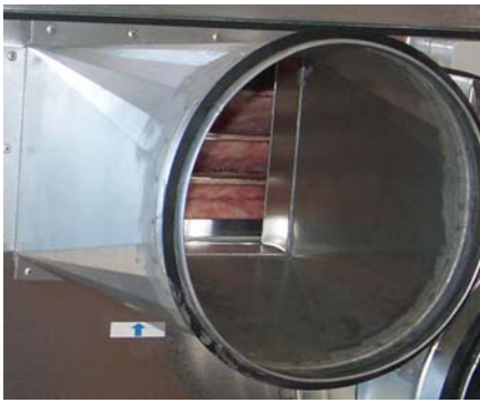
Adapter set OKM, suspension device and vibration dampers.
