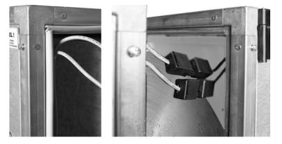
Fitting of the cooling section to other units is carried out using disc-lock, and assembly fittings for the largest; see details in the installation instructions for the unit.Parts for assembly are supplied with the unit and are found with other parts (drain trap, handle, etc.) in a box. It is important to make sure that the packing between the parts is in place and wires/plugs are not crushed. Snap-on connectors can also be connected together at the same time.
