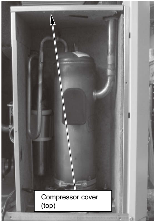
4. Remove the compressor cover (top).
