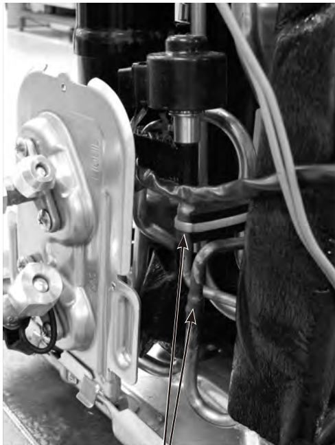
Brazed parts of LEV valve
