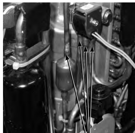
Brazed parts of 4-way valve
