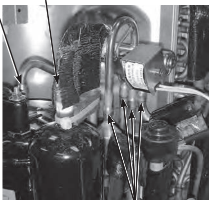
Brazed parts of 4-way valve
