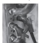
When fixing the indoor coil thermistor to the clip-shape/holder-shape part, the lead wire should point down.
