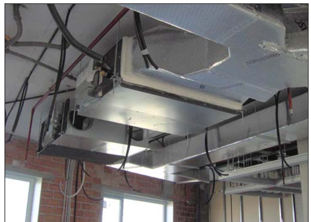
Lossnay units are suspended from ceiling.
