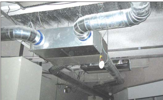
Lossnay installed in attic.
