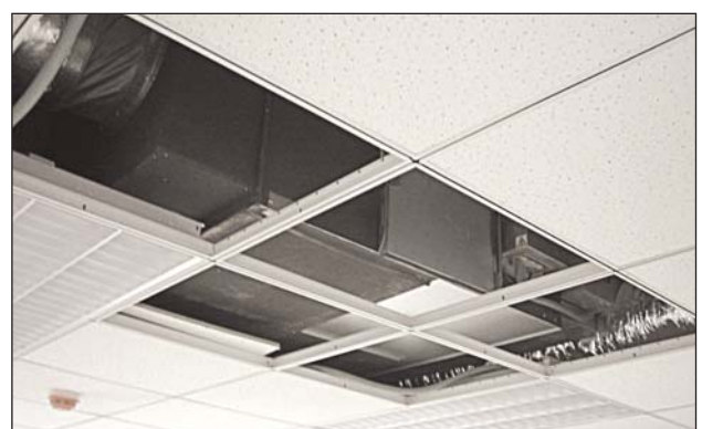
Lossnay installed in attic.
