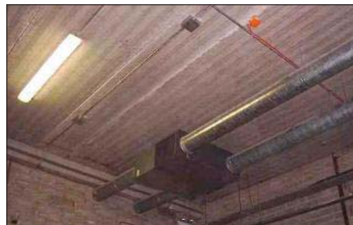
Lossnay unit is suspended from ceiling.
