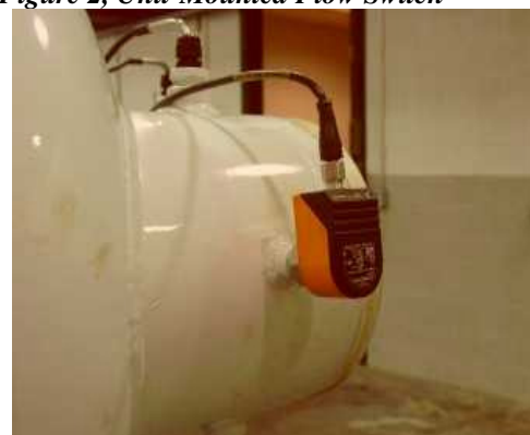
Figure 2, Unit-Mounted Flow Switch
