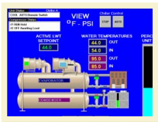
Figure 18, MicroTech II Control Panel
