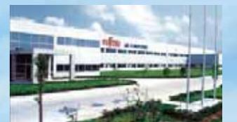
Fujitsu General (Shanghai) Co., Ltd.
