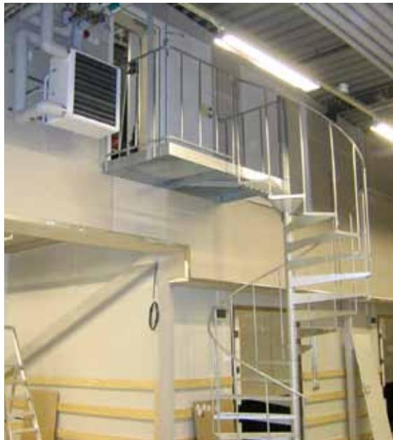
By turning the SWH, pipe connections are possible on both sides which makes it very easy to position. The air director, which has individually adjustable louvres directs the air flow as required.
