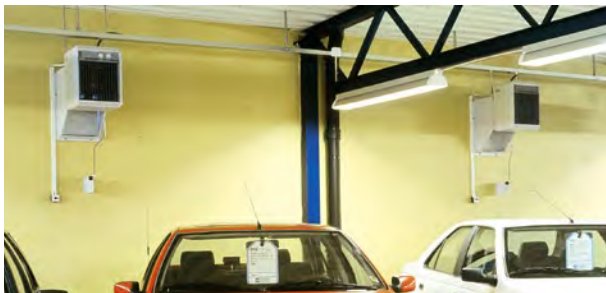
Mixing cabinets, available as an accessory, combine heating and ventilation. The mixing cabinet saves energy by mixing return air with fresh air in individually preset proportions.
