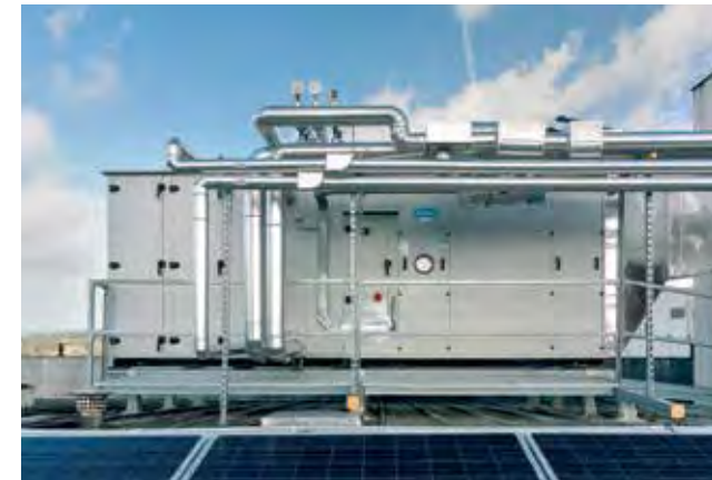
Figure 25: Example of an outdoor installation
