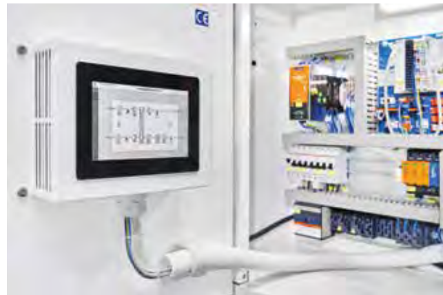
Figure 20: Examples of digital AHU control systems (image courtesy: TROX)
