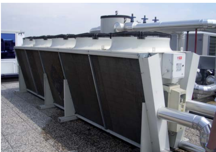
V-shaped roof-top dry cooler with 5 fans
